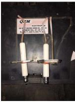
Replaced flame rod and ignitor due to poor condition.
